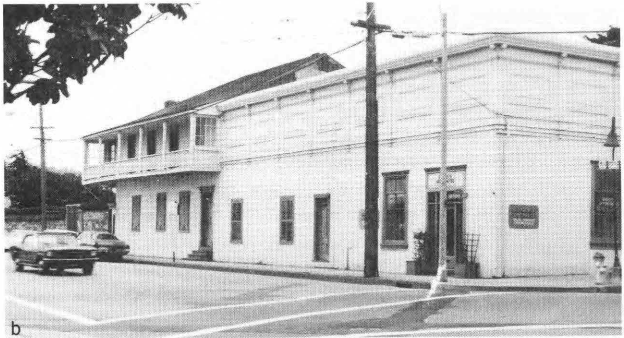
Figure 1. Cooper-Molera Adobe complex, Monterey, California: a) ca. 1870s. From left to right: John B. R. Cooper house (two story), Manuel Diaz home (with tile roof), Corner Store (signs and shingled roof); b) prior to beginning of restoration work in 1979. Victorian parapet obscuring earlier roof line has since been removed.
